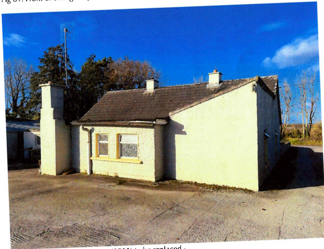
Fig 02. Existing rear extension (1961) to be replaced -
